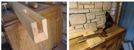
Figure 4: Cutting the Joinery
